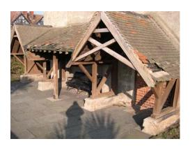
The historic perimeter brick and sandstone wall requires Ivy removal at various locations to the boundary with Victoria Drive and the Promenade. A structural engineer should assess the large vertical crack to the render at this junction. The flagged copings to 3No pillars at the vehicular access to the midden require replacement. The re-roofing of the feature Victorian shelters should be a priority.
